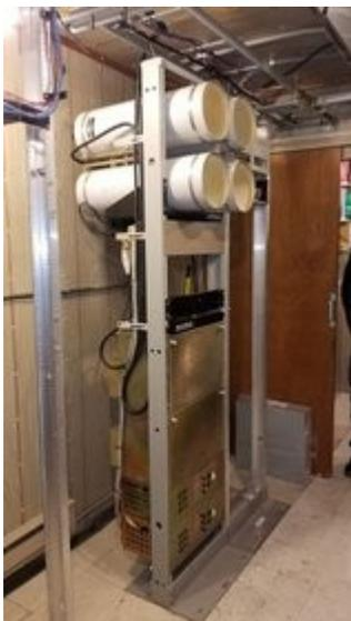
On 10 Sept., Paul N7PAS spent a good portion of the day out at Eric's shop removing the 90 equipment from the old cabinet and installing the repeater's components, duplexers and a power distribution panel in a 19 inch rack.
